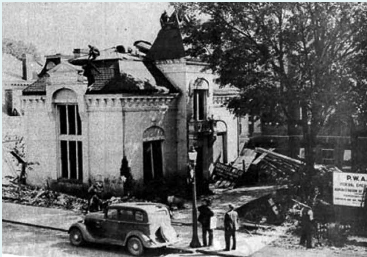
The courthouse of 1939 being torn down.
